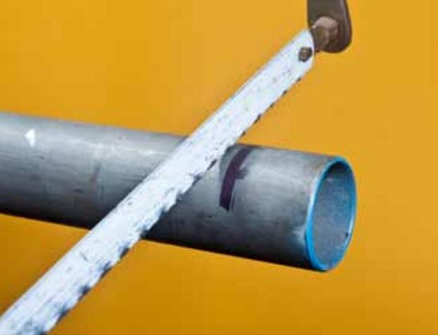
**4** Using a sharp hacksaw blade, cut the steerer 3-5mm below the line marked by the top of the stem to account for the space needed for proper bearing adjustment. Before making the cut it is worth holding the steerer up to the frame one last time to make sure the length still makes sense. Cut it straight and clean any burrs with a sanding block or flat file. A pipe-cutter can be used and ensures a straight cut but may require more post cut clean-up.
